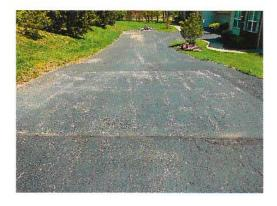
Periodic asphalt slurry sealing can help in the prevention of moisture penetration that can cause hairline cracking that eventually develops into alligatoring, potentially leading to an overall failure of the asphalt surface. As a further benefit, sealing helps to prevent the evaporation and loss of basic oils that bind the asphalt and allow for a pliable driving surface. This price also includes necessary striping.
