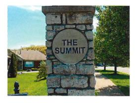
The entry monument is constructed of stone with a concrete cap and a concrete sign with engraved lettering. The monument measures 2' 8" x 2' 8" x 8' 6" (height). The sign is a 2' diameter circle.
